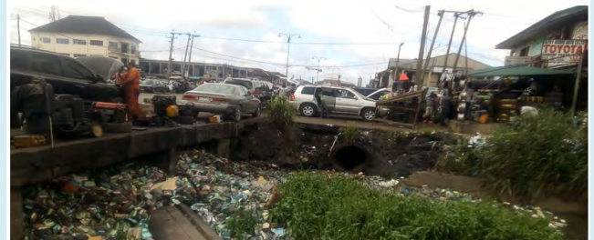
Figure 2: Wastes clogging stream channels at Ntawogba creek along Ikoku/Olu-Obasanjo Road.
